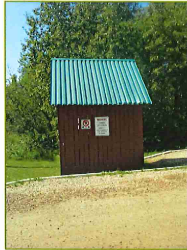
Figure 26. Tin roofing (above), asphalt shingles and treated wooden shakes are fire resistant when clean and clear of debris
